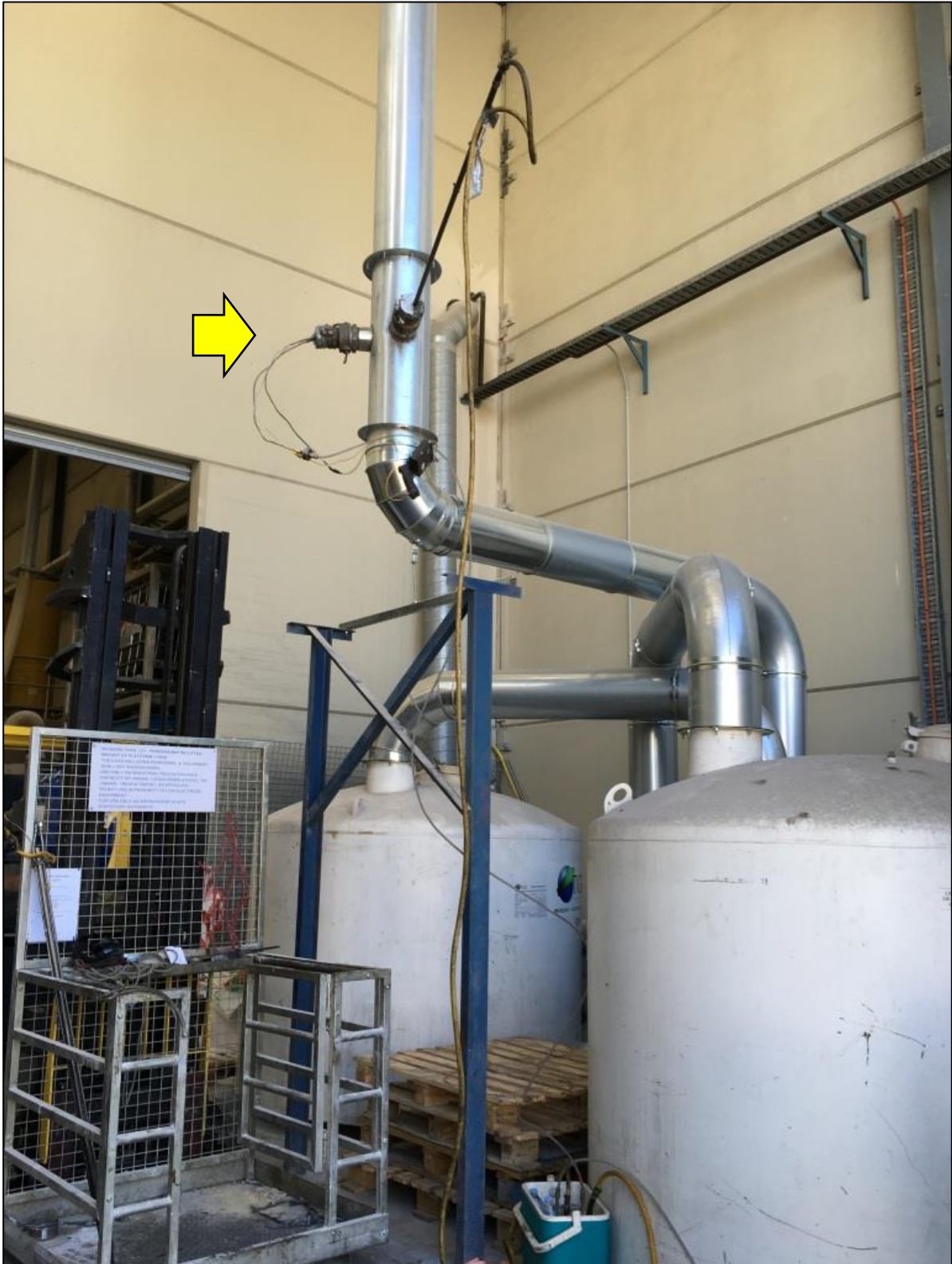
PHOTOGRAPH 1 DRY CARBON SCRUBBERS AND OUTLET SAMPLE PORTS
